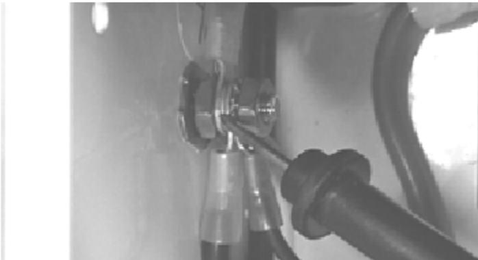
5. Check the voltage between the control box's chassis ground screw (on the left side wall) and the brass buss bar running across the top of the fuse block. If there is no voltage detected, check all connections.
